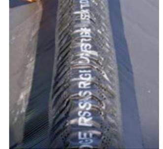
**3** Remove the tape protector and smooth the ridge roll over the laid tiles without crushing the corrugations.
