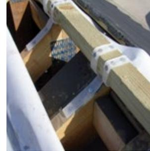
**1** Install the underlay 30mm down from the ridge apex and nail the ridge batten connectors to the roof rafters with two Galvanized Clout nails. Wrap the other legs around the 50 x 50mm ridge batten and secure with Galvanized Clout nails.
