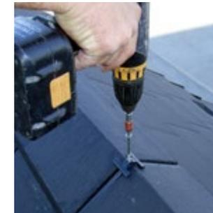
**5** Position the Fast Union Clip into the slot in the top of the Fast Union and secure with the Fast Drive Screw.
