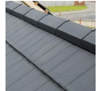
**6** Finish the ridge with either a block end ridge or ridge end cap from the dry verge system.
