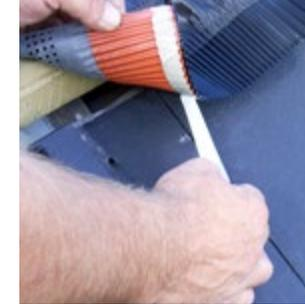
**2** Lay the roof tiles within specification. Place the fast Ridge Roll centrally over the tiles apex and nail the ridge batten connectors to the roof rafters with two Galvanized Clout nails. Wrap the other legs around the 50 x 50mm ridge batten and ensure the tiles are dust free and dry.
